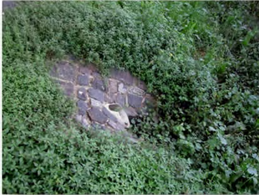
Outfall drain and stone apron at north end of Moonee Ponds Creek section, may contain early stone work
