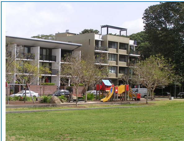
Example of higher density residential development overlooking a park setting.
